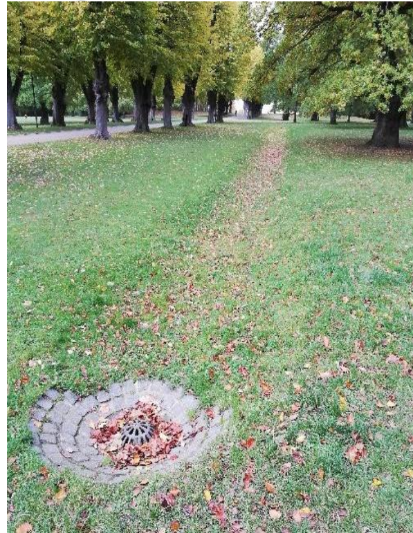
Figur 9. Svackdike i park
